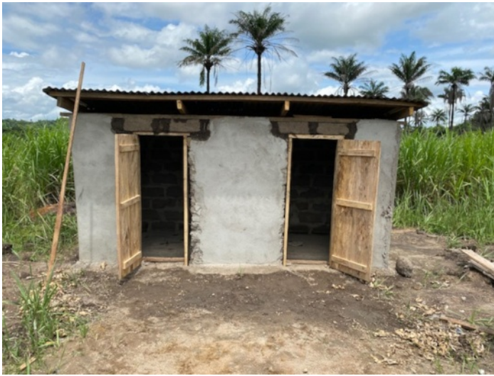
KDGO Toilet Project
