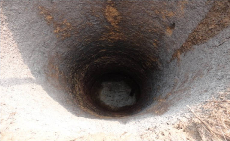
Digging in Progress( inside of the well)
